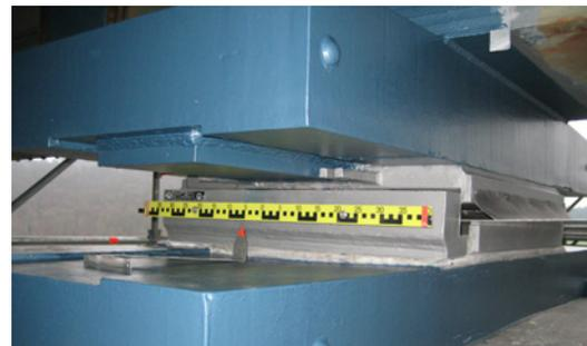
After: One of the first installed double cylindrical bearings at the Grenzwald bridge (A7 motorway).
