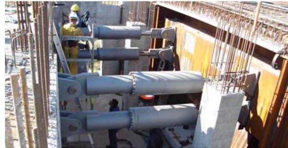
Fig. 31: Dampers (MHD) installed in a bridge
