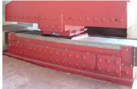
Fig.20 : Sliding isolator type SI
