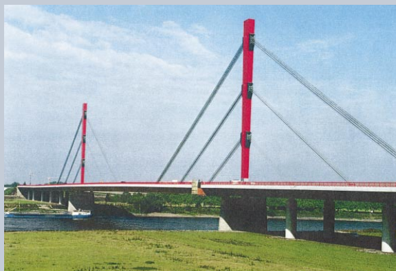
Bridge over the river Rhine at Beeckerwerth, Germany
