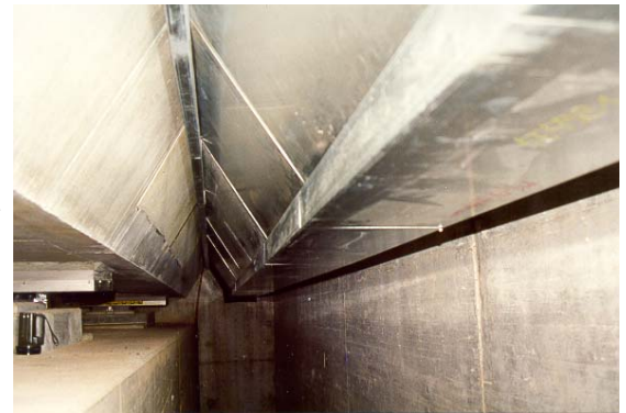
Readily mounted noise protection device (System A)
