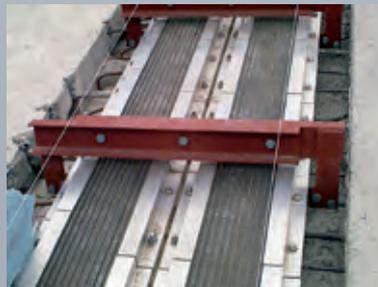
Conventional installation method, that is the prefabricated DB 160 expansion joint is lowered into an existing blockout and then concreted.
