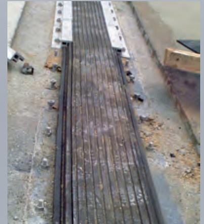
Alternative installation method. Here, the substructure is part of the precast segment, and the superstructure is fixed by means of shot bolts. This method requires no blockout and facilitates traffic on site.
